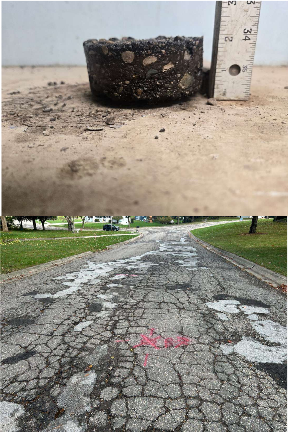
Core Photograph B-07: HMA Pavement = 2 inches
