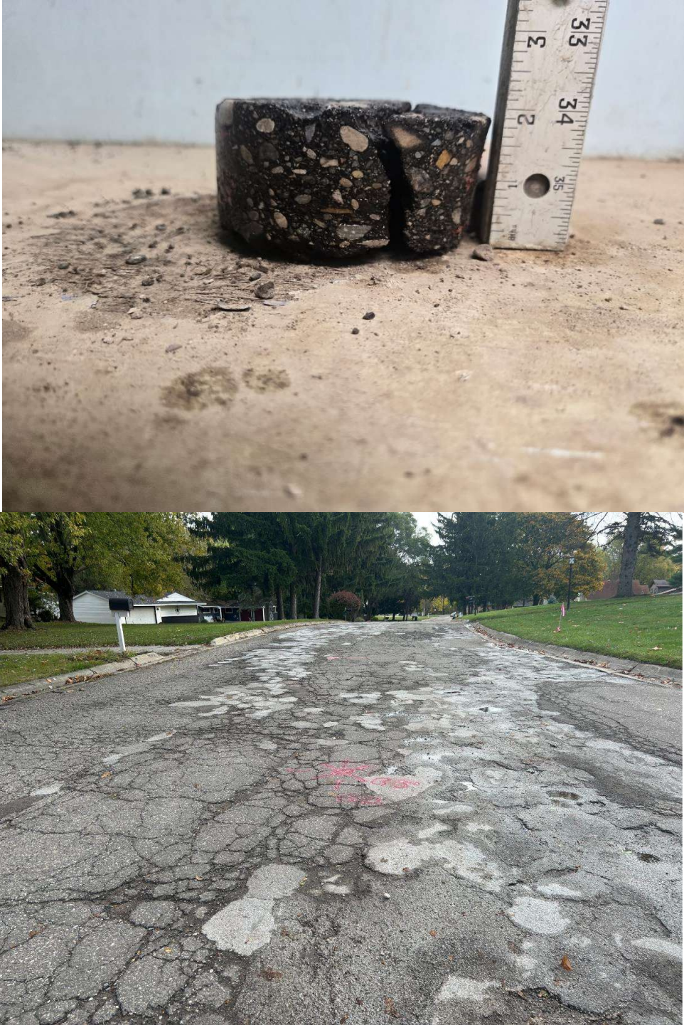
Core Photograph B-05: HMA Pavement = 2 inches
