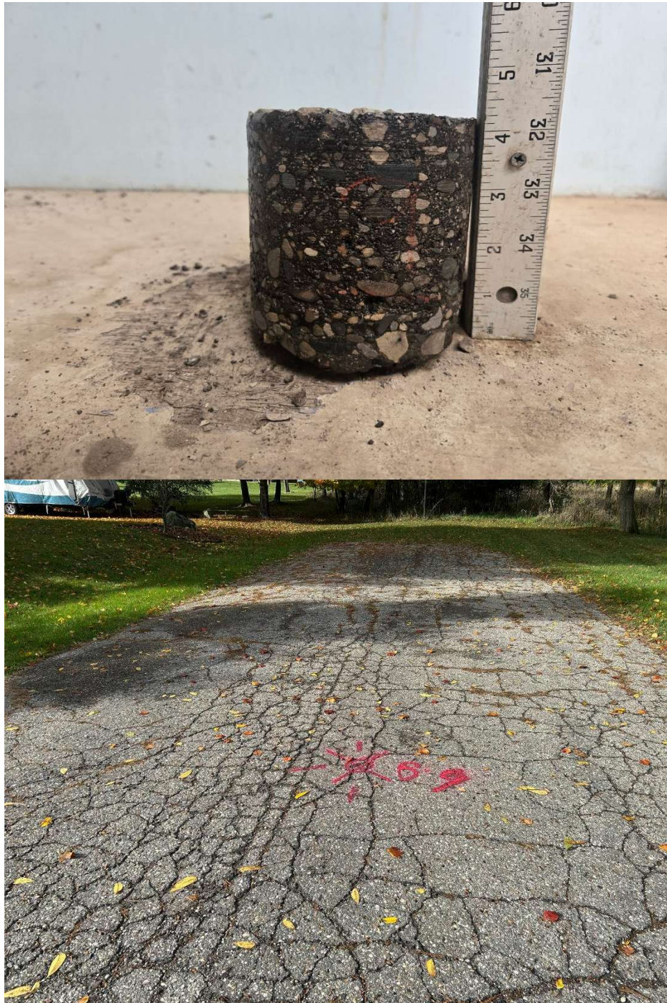
Core Photograph B-09: HMA Pavement = 4-1/4 inches
