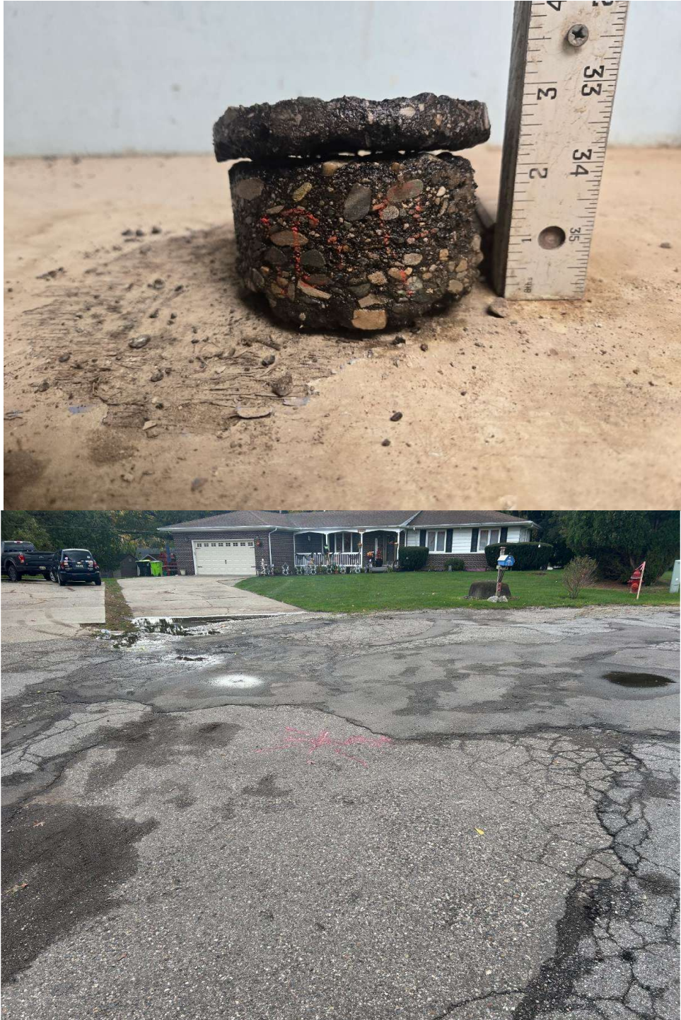
Core Photograph B-10: HMA Pavement = 3 inches
