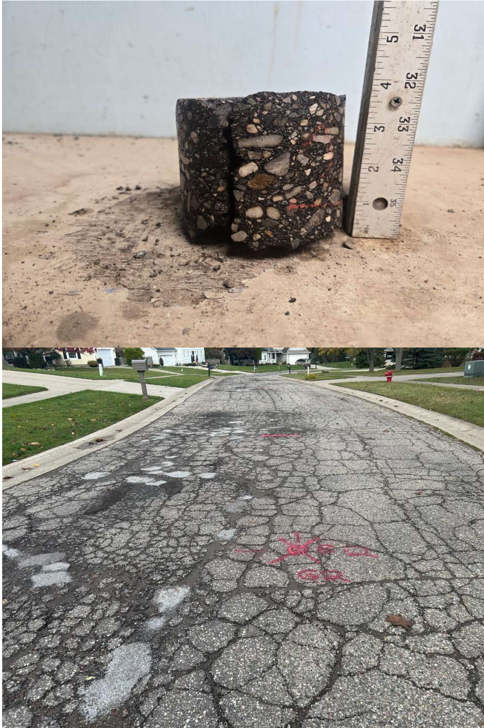
Core Photograph B-02: HMA Pavement = 3-1/2 inches
