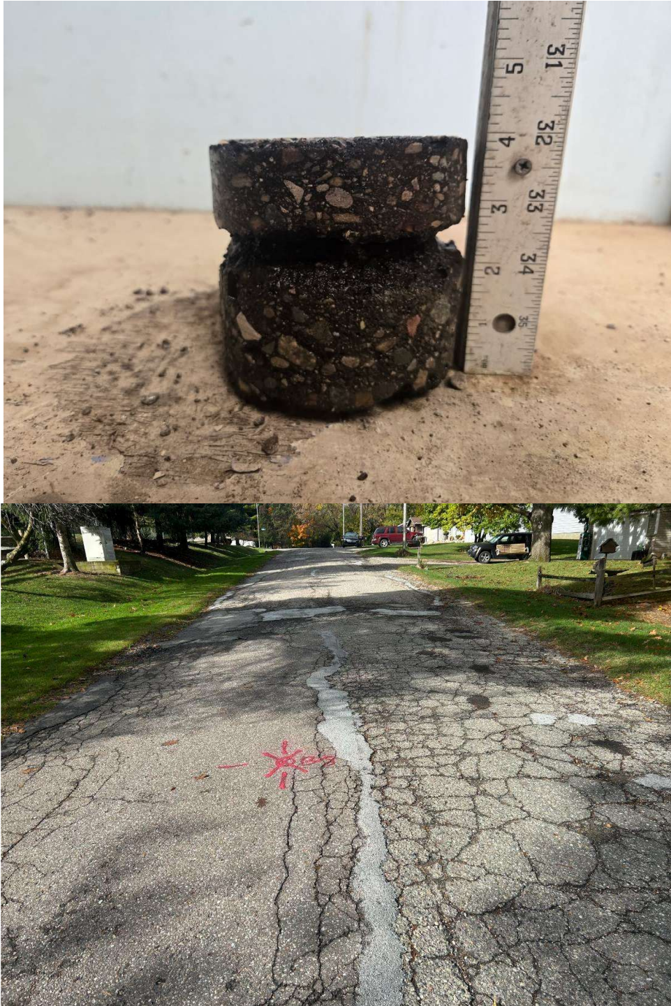
Core Photograph B-08: HMA Pavement = 4 inches
