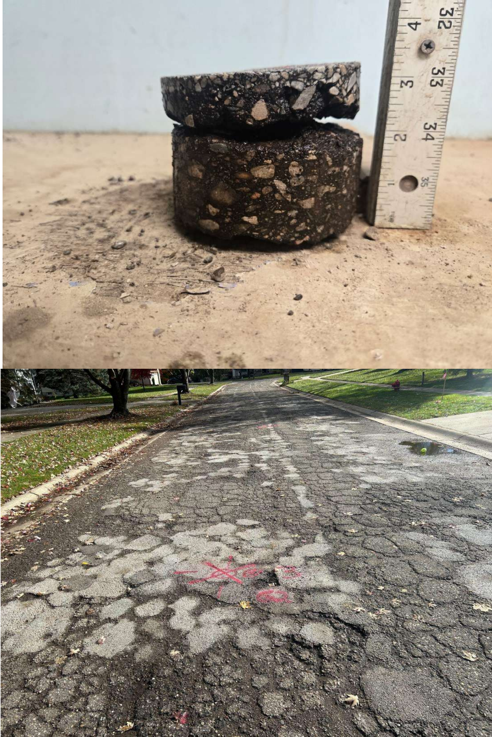
Core Photograph B-03: HMA Pavement = 3 inches
