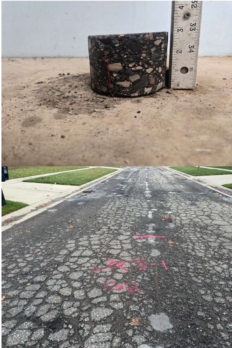
Core Photograph B-01: HMA Pavement = 2-3/4 inches
