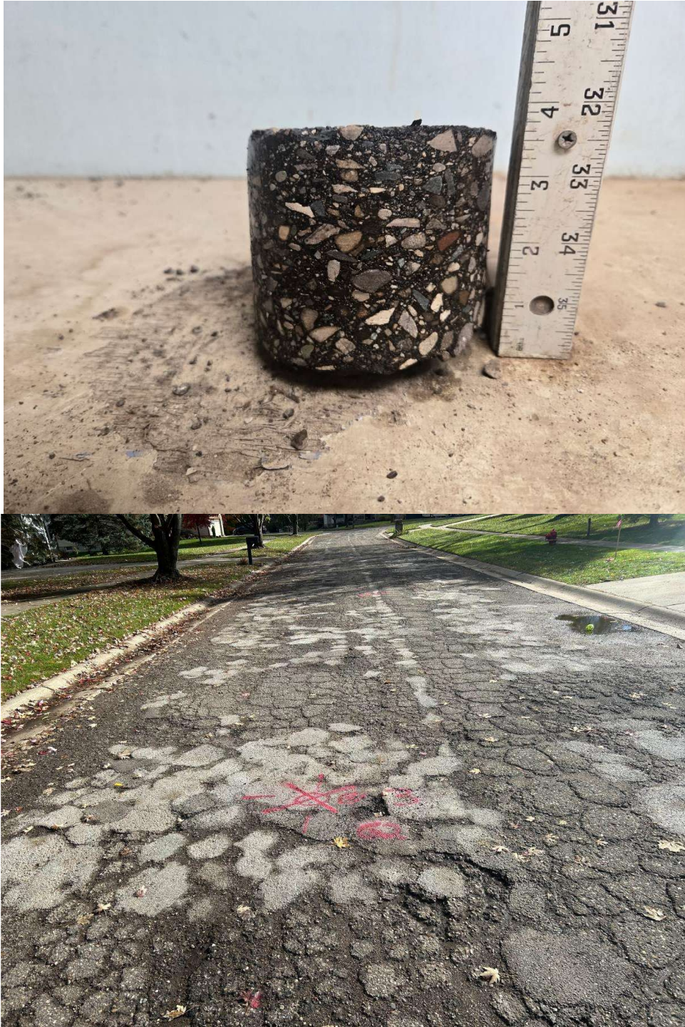
Core Photograph B-04: HMA Pavement = 3-1/2 inches
