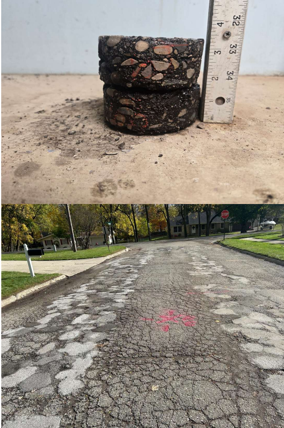
Core Photograph B-06: HMA Pavement = 3-1/2 inches
